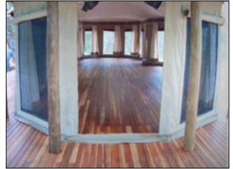
Tanzanian teak used in a decking application
